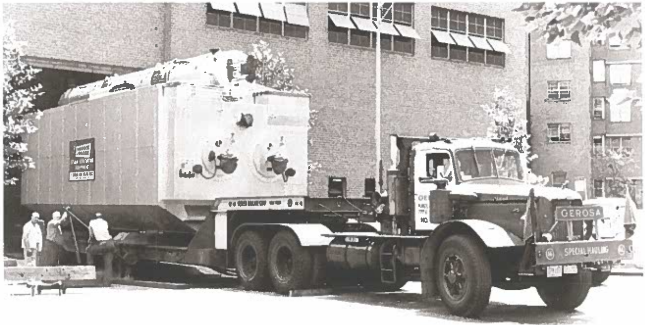
Installation of the original boiler for East River Housing circa mid-1950's
